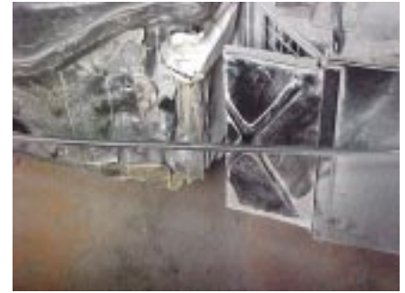
Cutting the air door for clearance
